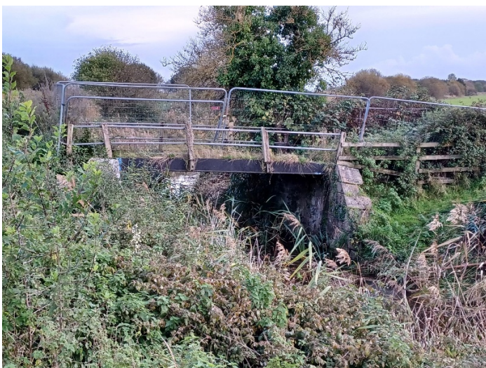
Current state of Bridge October 2023 point A on right of photo
