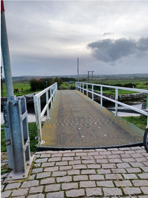
Point D looking back towards point C and Exminster in the distance.
