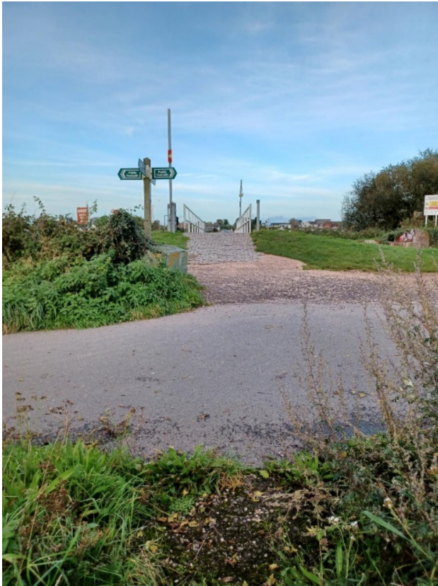
Point B looking towards C and over the bridge to point D and Topsham Ferry
